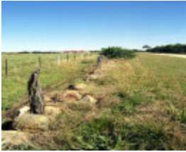
Dry Stone Wall J144
