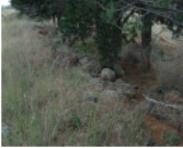
Dry Stone Wall J153
