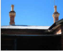
48-56 Taylor Street, chimney detail
