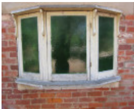
48-56 Taylor Street, detail of window added c.1920
