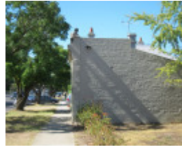
105 Lucan Street, side view
