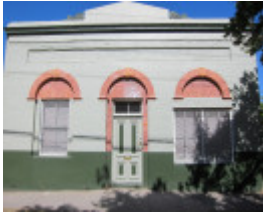
105 Lucan Street, shopfront
