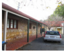
4 & 4A Weeroona Avenue, former bakery
