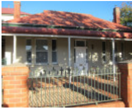
4 & 4A Weeroona Avenue, residence at front of site
