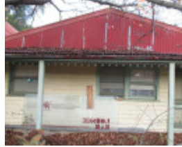
4 & 4A Weeroona Avenue, residence at rear of site
