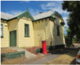
532 Napier Street, former White Hills Reading Rooms & Free Library
