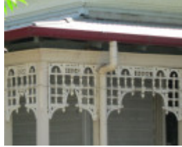
545 Napier Street, detail of cast iron frieze
