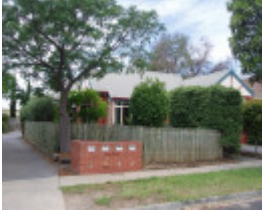
11/13 Meakin St, Geelong East
