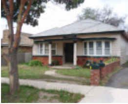
17 Meakin St, Geelong East
