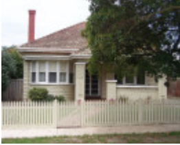
21 Meakin St, Geelong East
