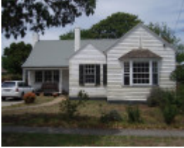
23 Meakin St, Geelong East
