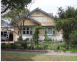
25 Meakin St, Geelong East
