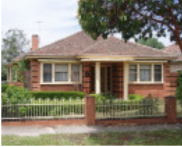
29 Meakin St, Geelong East
