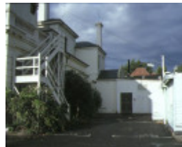
frognall mont albert road canterbury side stairway
