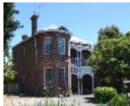
Photo 6: Brooklyn, principal (east) elevation, November 2015.
