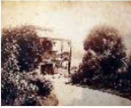
Figure 12: 'Newtown Brae', east elevation (north wing), n.d. [c.1900]. Source: Jan Phelan, Welshpool.
