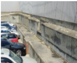
Retaining wall and raised platform (Element 7)
