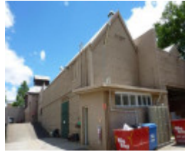
Building 4, looking west; the entry to Building 3 is to the right of the picture
