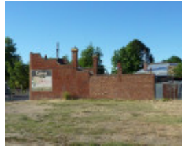
Property as viewed from the north
