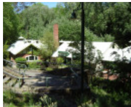
H2098 Hepburn Mineral Springs Reserve_bathhouse_Nov.05
