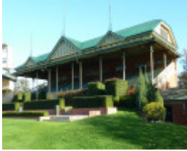
The 1902 Grandstand as viewed from the east
