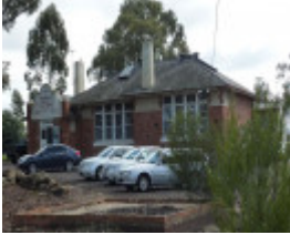
The main building of the former Bendigo East school, viewed from the east
