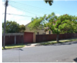
Photo 3: Garage outbuilding, 31 Nantes Street, 2015.
