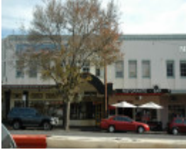
58 Moorabool Street, Geelong
