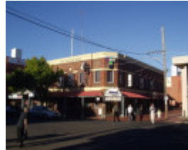
Wool Exchange Hote - 59 Moorabool Street, Geelong - Photo 2
