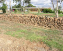
Dry Stone Wall N226 - Sinclairs Road Boundary
