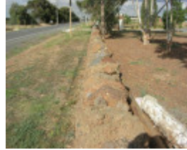
Dry Stone Wall N226 - Sinclairs Road Boundary
