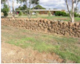
Dry Stone Wall N226 - Sinclairs Road Boundary
