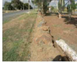
Dry Stone Wall N226 - Sinclairs Road Boundary
