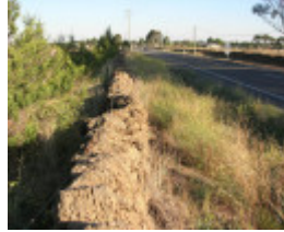
Dry Stone Wall N240 - Sinclairs Road Boundary
