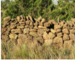
Dry Stone Wall N240 - Sinclairs Road Boundary
