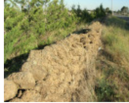
Dry Stone Wall N240 - Sinclairs Road Boundary
