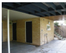
2017, below rear deck.JPG
