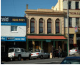
189 Moorabool Street, Geelong
