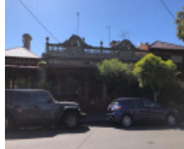
64-74 Upton Road, Windsor
