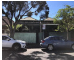
64-74 Upton Road, Windsor
