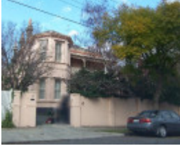
15 Moorehouse Street, Armadale
