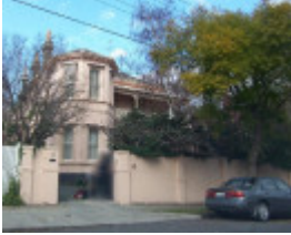
15 Moorehouse Street, Armadale
