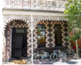
612 Malvern Road, Prahran
