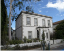
52 Albion Street, South Yarra
