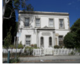
52 Albion Street, South Yarra
