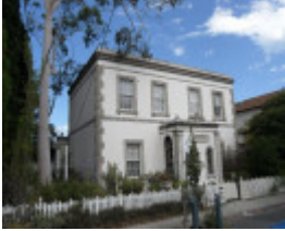
52 Albion Street, South Yarra
