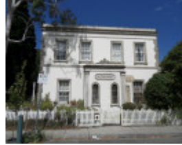
52 Albion Street, South Yarra
