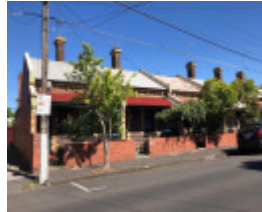
49-59 Upton Road, Windsor
