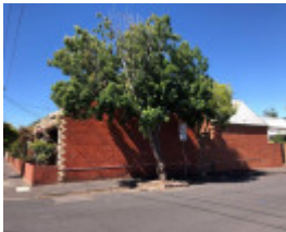
49-59 Upton Road, Windsor
