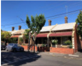
49-59 Upton Road, Windsor
