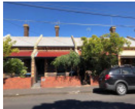
49-59 Upton Road, Windsor
