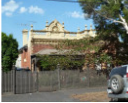
56 Stanhope Street, Malvern
