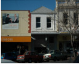
209 Moorabool Street, Geelong
