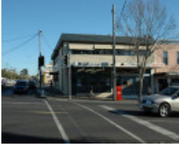
210 Moorabool Street, Geelong
