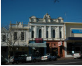
215-217 Moorabool Street, Geelong
