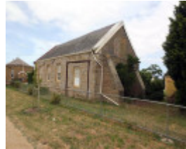
Photo 2: Former Church building, north & west elevations, 2016.
