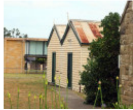
Photo 3: Former Sunday School, east elevation, 2016.
