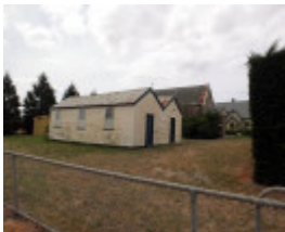
Photo 4: Former Sunday School (middle ground) & Church (background), south elevations, 2016.
