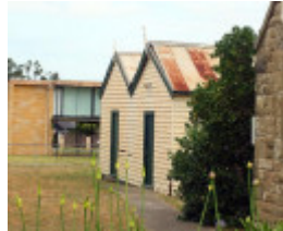
Photo 3: Former Sunday School, east elevation, 2016.
