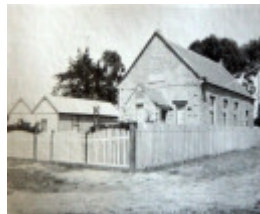
Figure 4: T. Holmes, Ceres Wesleyan Methodist Church and Sunday School, looking from intersection of McCann & Wheatsheaf Streets, c.1930. Source: T.T. Holmes photograph collection, c/o David Rowe.
