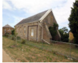
Photo 2: Former Church building, north & west elevations, 2016.
