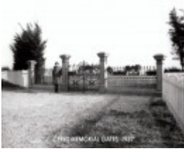
Figure 5: Ceres Memorial Gates, 1937, with Alfred Beaumont "Mont" McDowall standing. Also note the early pavilion in the background built in 1913 (left of central gate bay), gum and cypress trees forming the perimeter of the reserve & the timber picke
