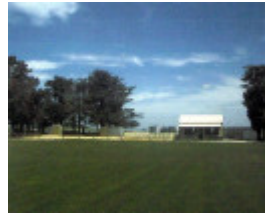
Figure 9: Barrabool Recreation Reserve looking south to the pavilion following alterations, n.d. [c.2014]. Source: Crown Reserve file Rs 4144 DELWP.
