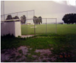
Figure 8: Barrabool Recreation Reserve looking south to the pavilion prior to alterations & additions, 14 August 1996. Source: Crown Reserve file Rs 4144 DELWP
