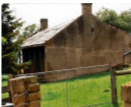
Figure 7: J.T. Collins, 'Barwonside', front and south elevations, 1993. Source: G. Dekker, A. Greenwood & S. Taylor, 'Perspectives on Ceres', architectural conservation report, School of Architecture, Deakin University, 1993, p.45.
