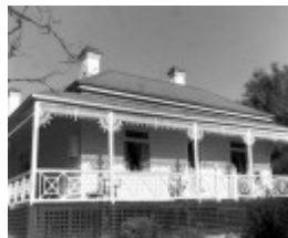
Figure 6: 'Erinvale', 285 Gully Road, 1997. Source: David Rowe.
