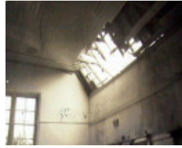
Figure 7: Interior, Ceres State School showing roof damage, 6 December 1948. Source: VPRS 10516/P3 Unit 7 Public Record Office Victoria.
