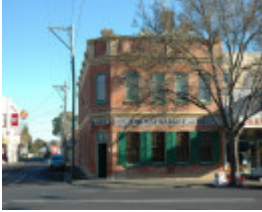
244 Moorabool Street, Geelong
