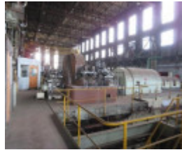
Wet Section Building
