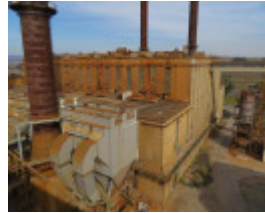
View south from the top of No.1 Briquette Factory looking at power station.
