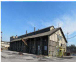
View southwest to Briquette Storage Shed.
