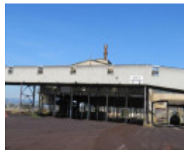
View south to briquette loading station.
