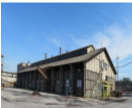
View southwest to Briquette Storage Shed.
