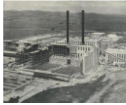
Morwell Briquette Works under construction, 1959.
