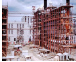
Construction of the Briquette Factories, undated.
