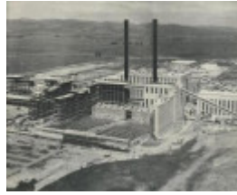
Morwell Briquette Works under construction, 1959.
