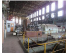
Wet Section Building
