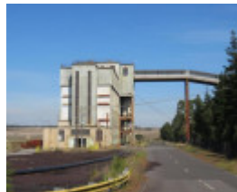
View south to the raw coal bunker and conveyor.
