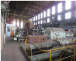
View inside the Turbine House, looking northeast.
