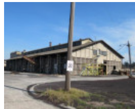
Briquette Storage Shed
