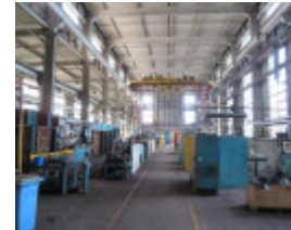
View inside the Mechanical Workshops, looking east.
