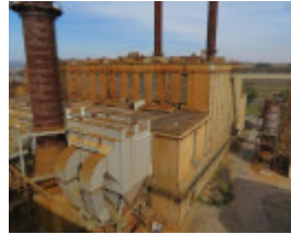
View south from the top of No.1 Briquette Factory looking at power station.
