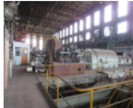
Wet Section Building
