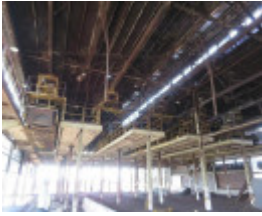
View from under the briquette loading station.
