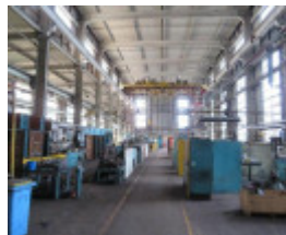
View inside the Mechanical Workshops, looking east.
