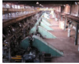
View of briquette machinery in No.1 Briquette Factory, looking east.
