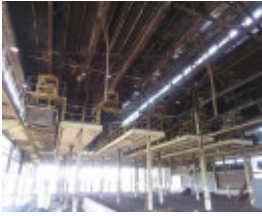
View from under the briquette loading station.
