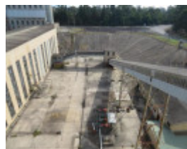
View east from the top of No.1 Briquette Factory looking at the conveyors and North West Corner Station.
