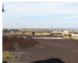
View east towards the briquette storage area, with the location of the former No.1 cooling tower in the middle, and the briquette storage shed in the background.
