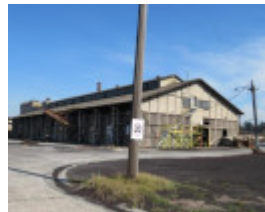
Briquette Storage Shed
