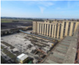
View northeast from the top of No.1 Briquette Factory looking at side of the Briquette Factory (right) and the collecting and feeding conveyors (left)
