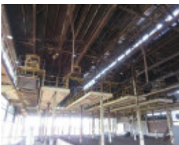
View from under the briquette loading station.
