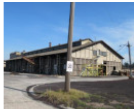
Briquette Storage Shed
