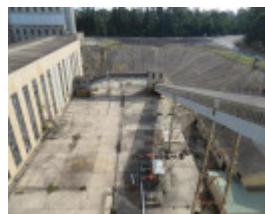
View east from the top of No.1 Briquette Factory looking at the conveyors and North West Corner Station.
