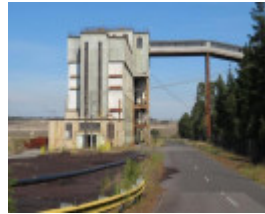
Raw Coal Bunker
