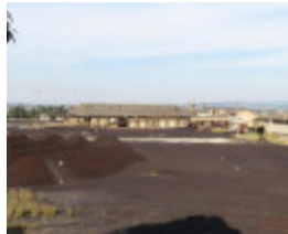
View east towards the briquette storage area, with the location of the former No.1 cooling tower in the middle, and the briquette storage shed in the background.
