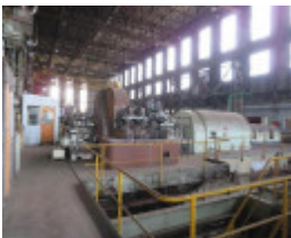
View inside the Turbine House, looking northeast.
