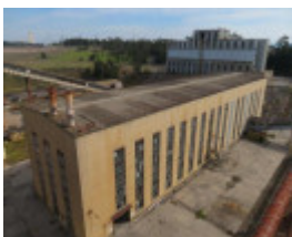
View southwest from the top of No.1 Briquette Factory looking at Wet Section No.1 building (foreground) with the raw coal bunker visible (background)
