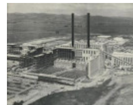
Morwell Briquette Works under construction, 1959.
