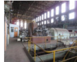
Wet Section Building
