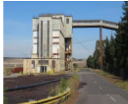
Raw Coal Bunker
