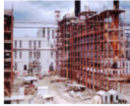
Construction of the Briquette Factories, undated.
