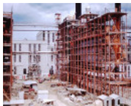
Construction of the Briquette Factories, undated.
