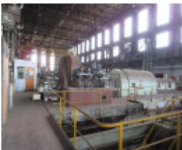
View inside the Turbine House, looking northeast.
