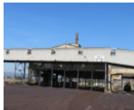
View south to briquette loading station.
