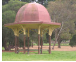
H2095 Eastern Park 29 10.2005 Former Ladies Kiosk
