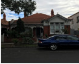
51 King Street FITZROY NORTH
