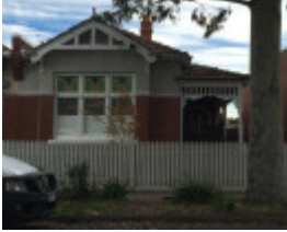
49 King Street FITZROY NORTH
