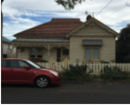
45 King Street FITZROY NORTH
