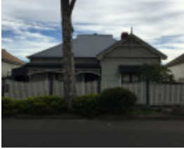
43 King Street FITZROY NORTH
