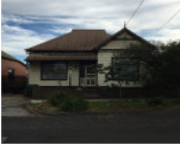
39 King Street FITZROY NORTH
