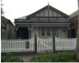
35 King Street FITZROY NORTH
